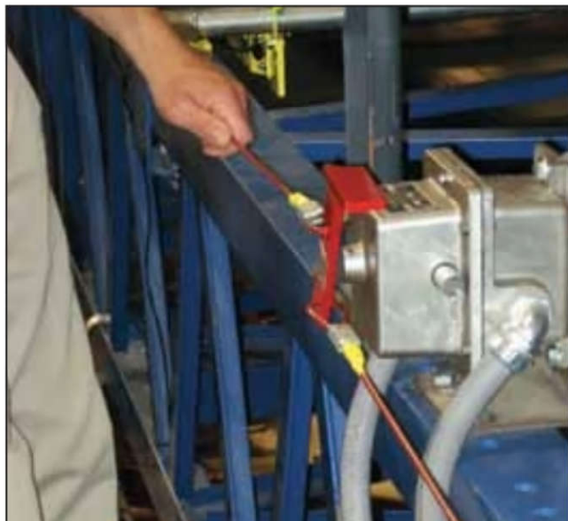
Figure 18 Emergency stop, pull-cord type
