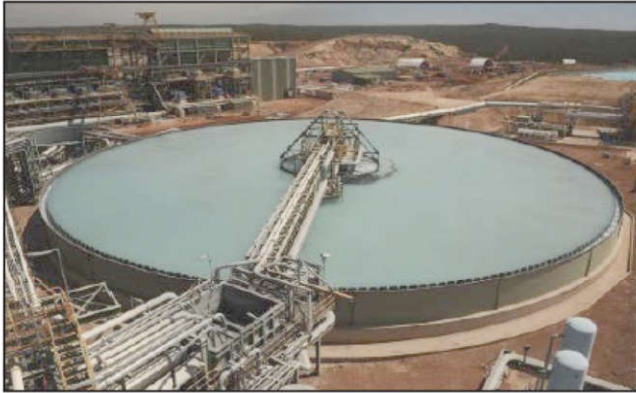
Figure 11 On-ground tank with concrete floor and bolted steel walls
