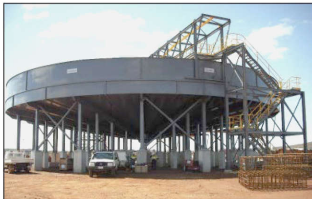
Figure 10 Elevated thickener tank with bolted steel construction
