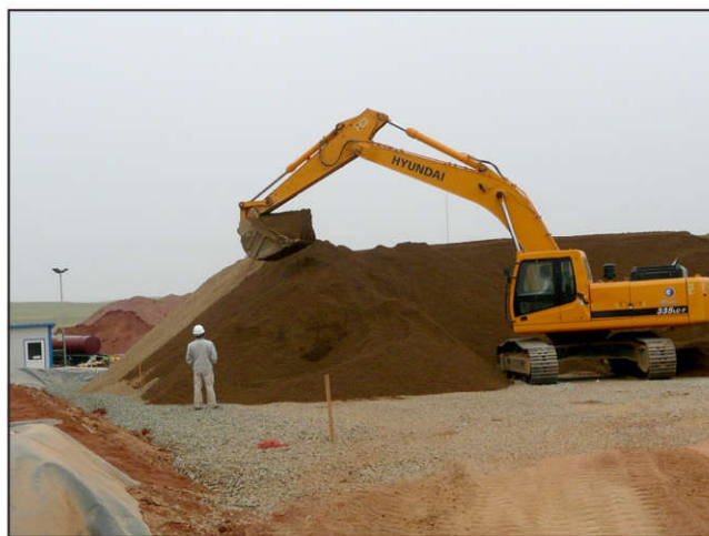
Figure 8 Excavator stacking a 5-m (16-ft) heap
