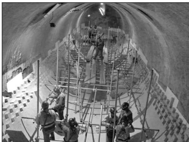
Figure 21 Pressure vessel refractory lining installation in progress
